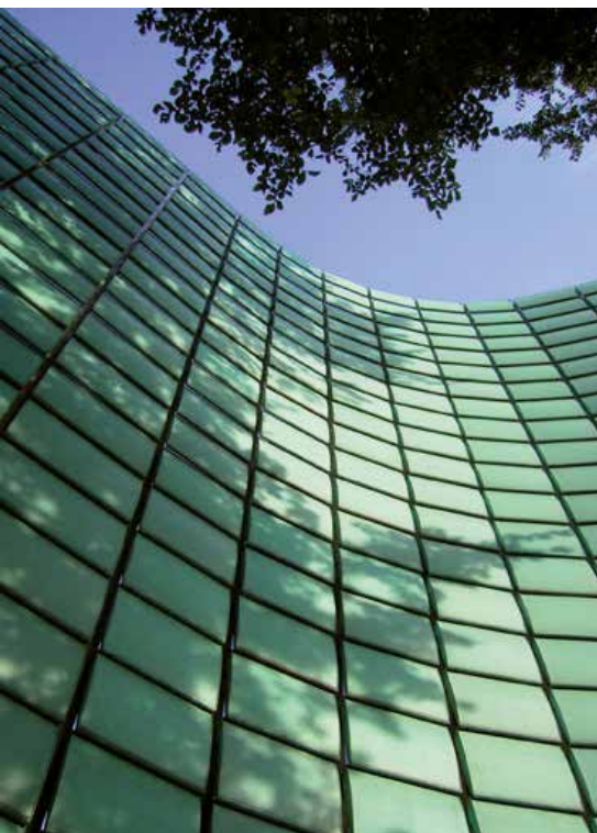
Danish Embassy, Berlin, clad with oxidised copper plates.
